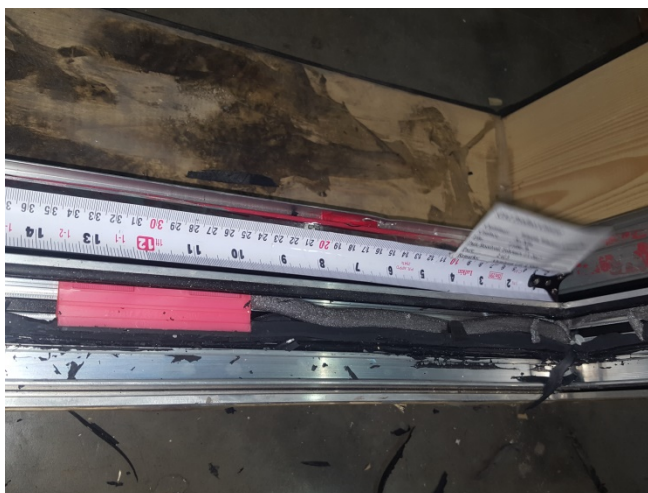
Figure 6: Silicone bead and foam backer rod, setting block assembly at bottom rail.
