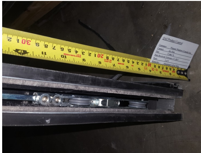
Figure 16: Rollers at bottom of active slab, interlock-side corner.
