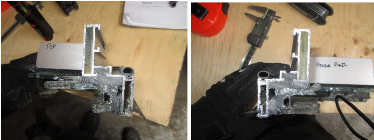
Casement Sash Profile – Latch Rail, Left; Bottom Rail, Right
